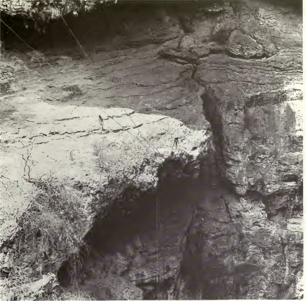
Plate 2. A close-up of the arrowed area in Plate 1 to indicate the size of the sink hole.
